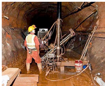
Figure 2: Workers drill a core to take stress-measurements in order to evaluate the quality of the rock for construction of very large caverns. The caverns will be part of the Sanford Lab and will continue to house DUSEL experiments. (Steve Babbitt, Black Hills State University/ SDSTA)
